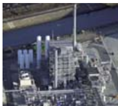
Air Products' reformer in Carson feeds refineries.
